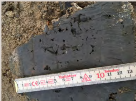
Example of channels within bentonite sealing
